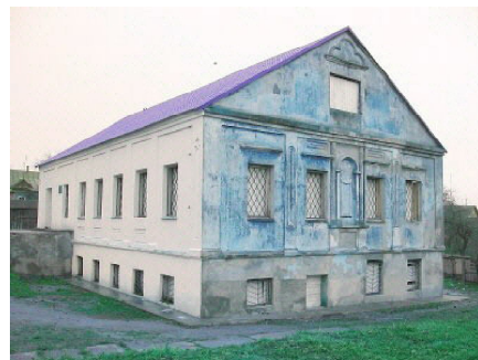
The Yeshiva building today
